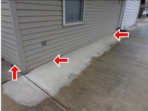
2.0 Picture 1 left side and rear ground contact
