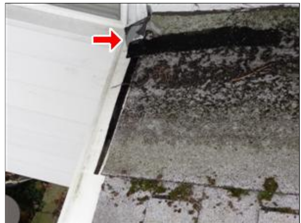
1.0 Picture 9 patch work at gutter rear of home
