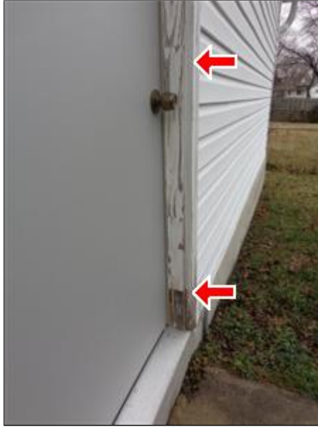
2.0 Picture 4 rear garage door
