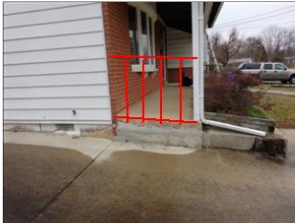
2.3 Picture 1 add handrail or steps
