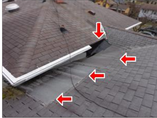
1.0 Picture 5 rolled roofing this area
