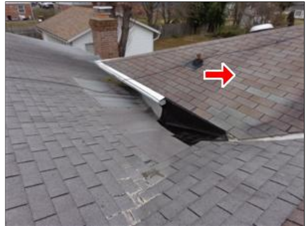
1.0 Picture 2 newer main roof
