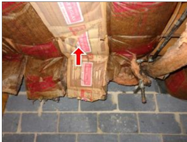
5.0 Picture 2 paper should be against floor
