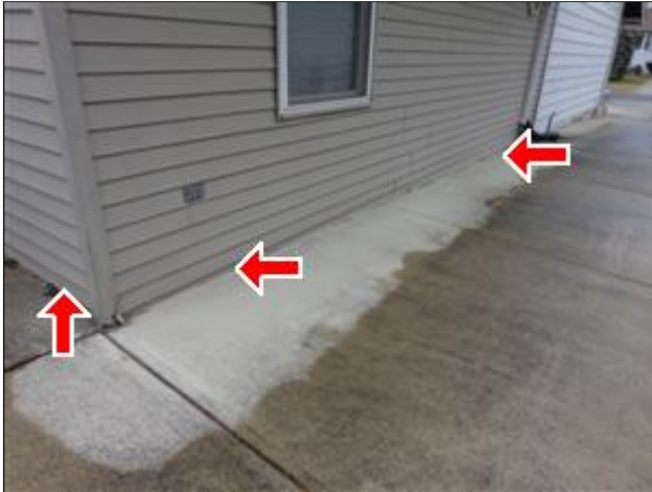
2.0 Picture 1 left side and rear ground contact
