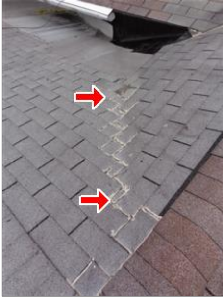
1.0 Picture 4 repairs to valley
