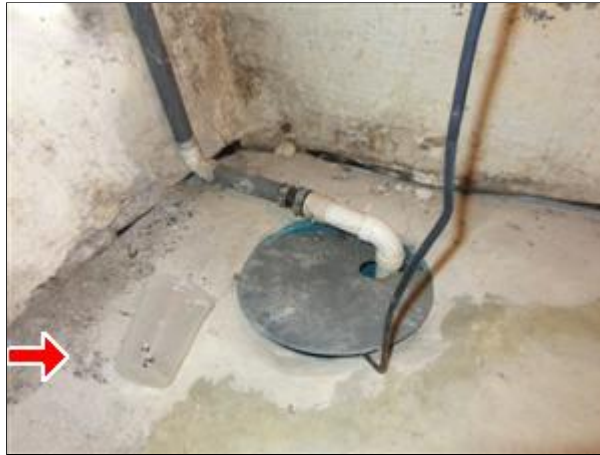
5.0 Picture 1 drain tile under floor
