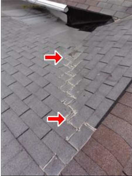
1.0 Picture 4 repairs to valley
