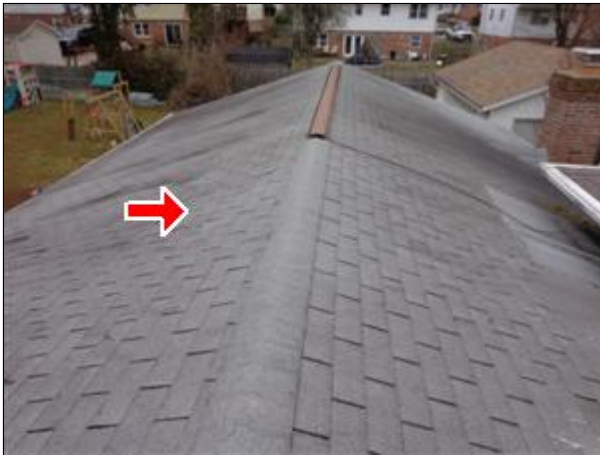
1.0 Picture 1 older addition roof
