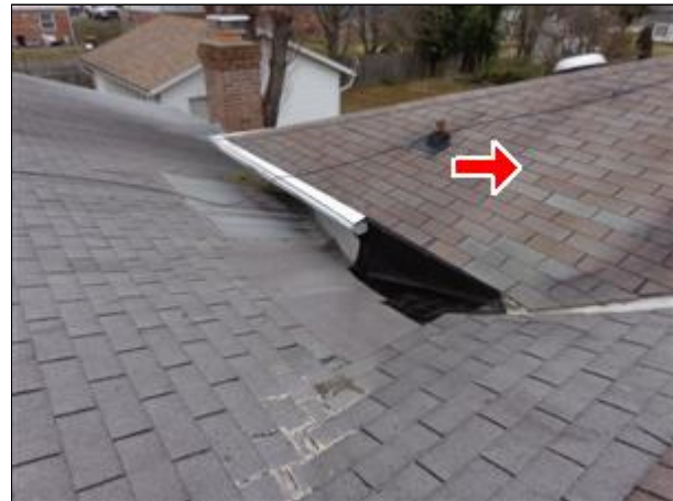
1.0 Picture 2 newer main roof
