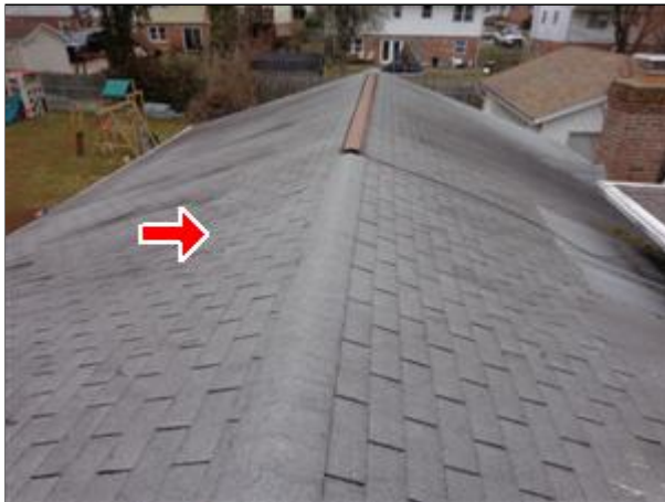
1.0 Picture 1 older addition roof
