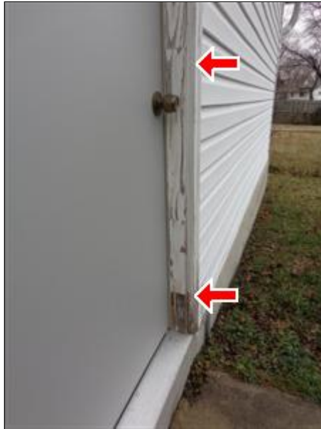
2.0 Picture 4 rear garage door
