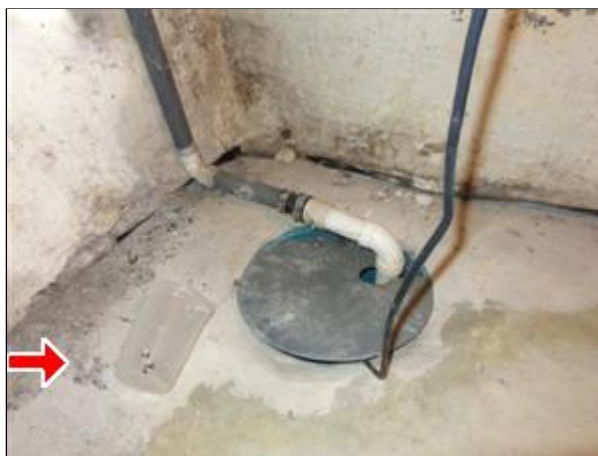
5.0 Picture 1 drain tile under floor
