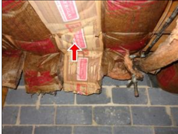
5.0 Picture 2 paper should be against floor
