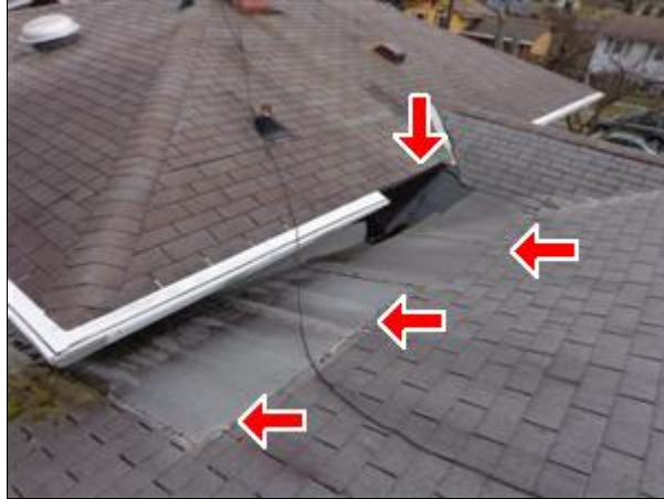
1.0 Picture 5 rolled roofing this area
