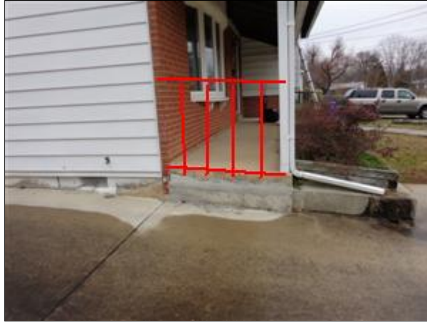
2.3 Picture 1 add handrail or steps
